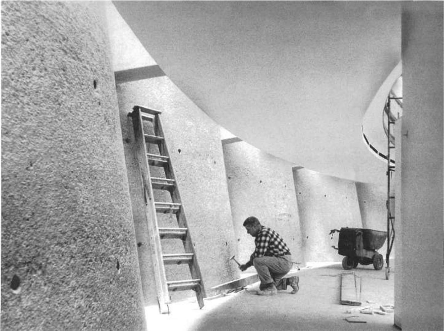
**Figure 34: Temple Beth Zion – Building Construction; workman finishing interior concrete walls
